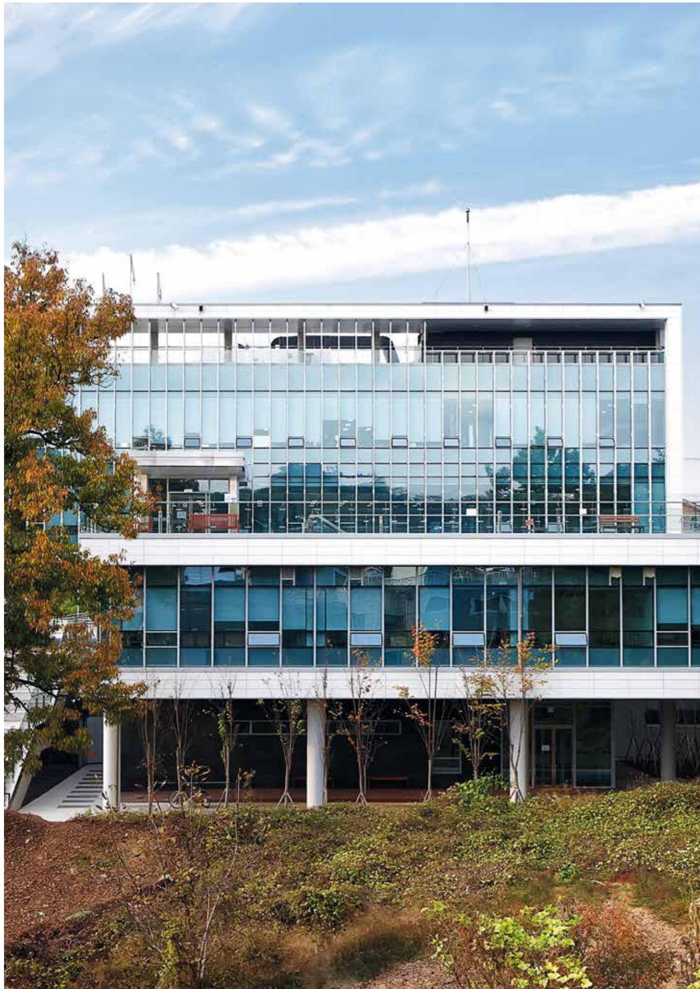
tempio®[projects] Jan Dang Library, South Korea
