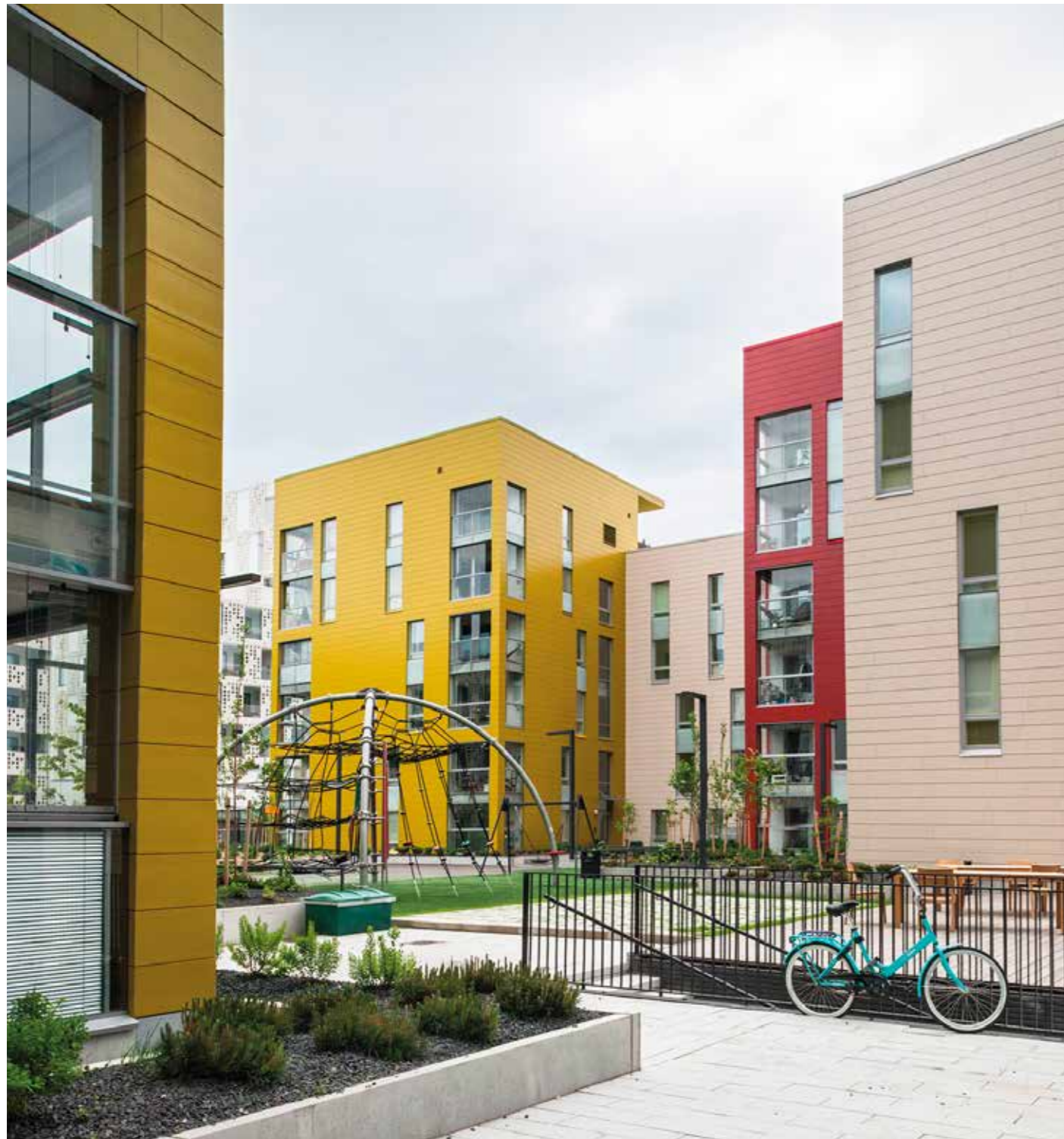
tempio® [projects] Saukonkanava, Helsinki, Finland.
